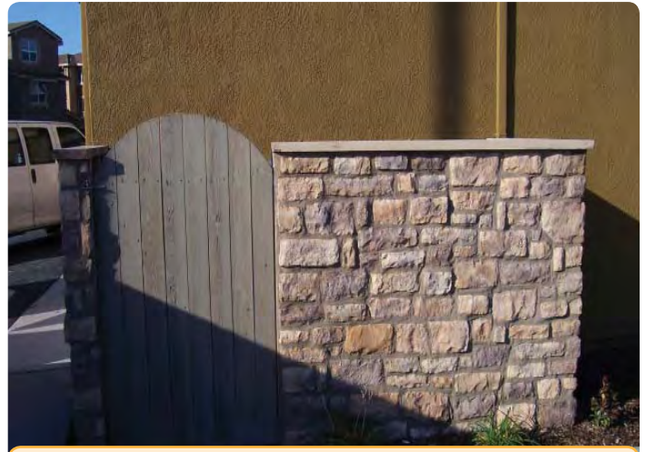
Utility meters effectively screened from view.
