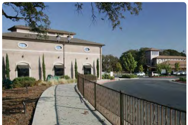
Wrought iron fencing maintains visual connectivity with open space.
