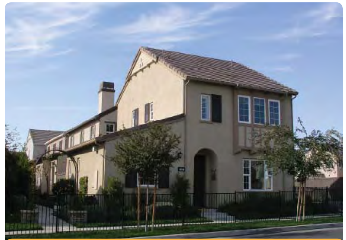
Garage placement in the alley bring living areas closer to the street.
